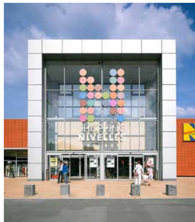
Centre commercial, Nivelles
