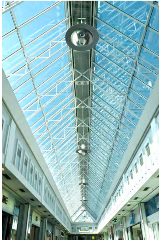
Picture: solar film and start up roof renovation
