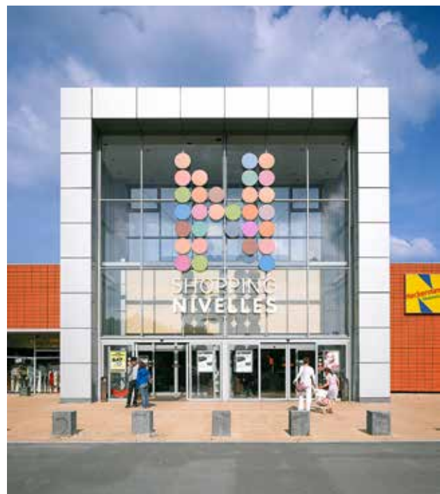
Centre commercial, Nivelles
