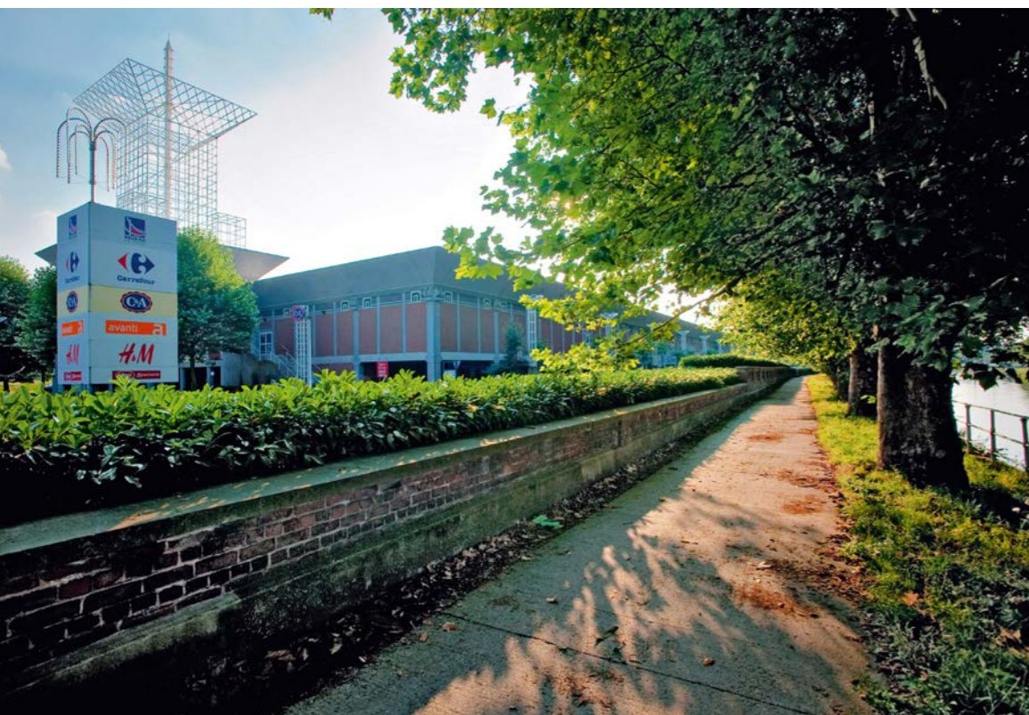
Centre commercial Belle-Ile, Liège
